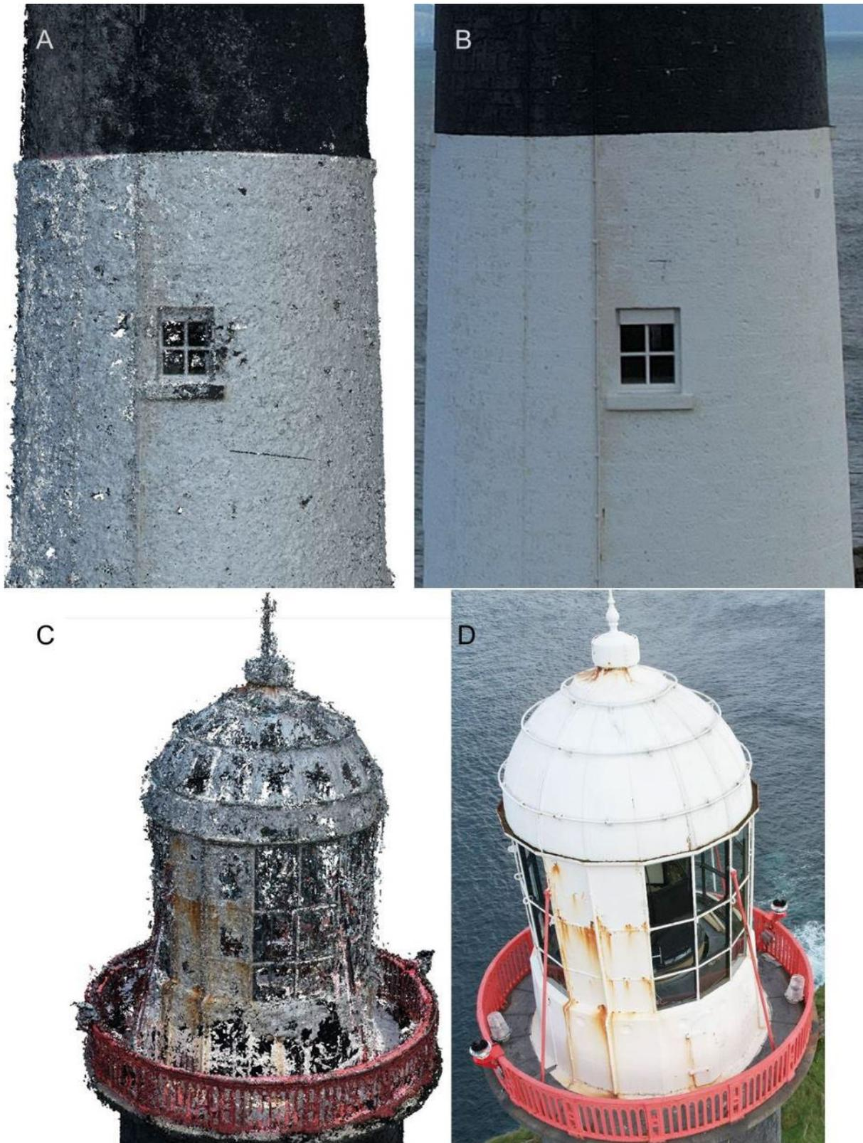
Figure 16: Close up view of the dense cloud showing the edge points and errors from on the mid-section of the lighthouse (A) and a corresponding photo (B) and errors at the top of the lighthouse (C) and corresponding photo (D)
